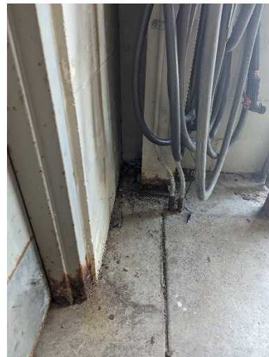
Fig 6. Corrosion at steel column base
