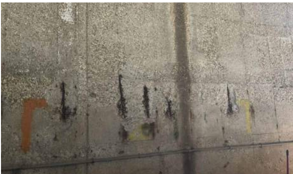
Exposed Rebar
