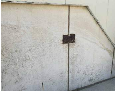
Corroded Connection of Precast Panels
