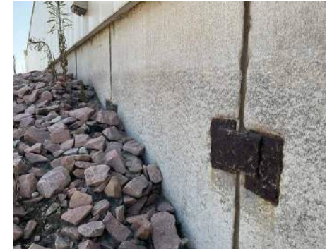
Rock Piles and Corroded Connections 2
