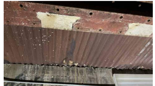
Steel Floor Beam and Deck/Close View
