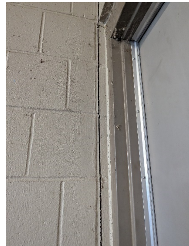
Fig 2. Separation of CMU at wall intersection
