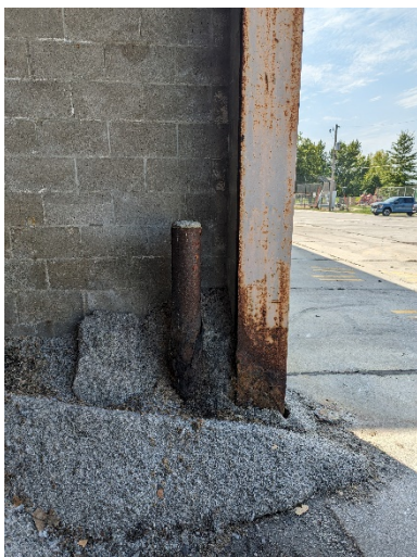
Fig 15. Corrosion at steel jamb posts and bollards
