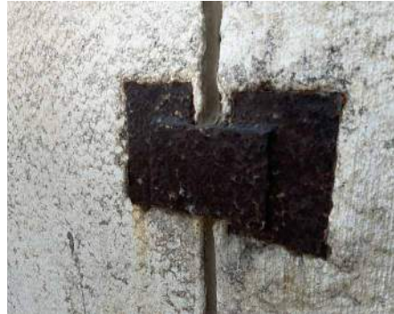
Corroded Connection of Precast Panels
