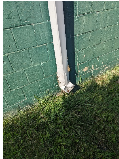
Fig 8. Damage to downspout
