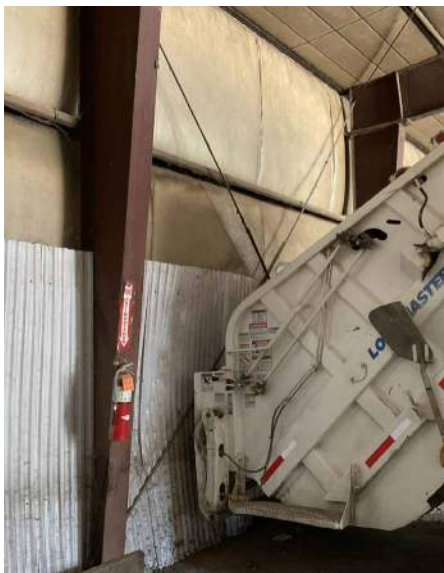
Damaged X-Bracing
