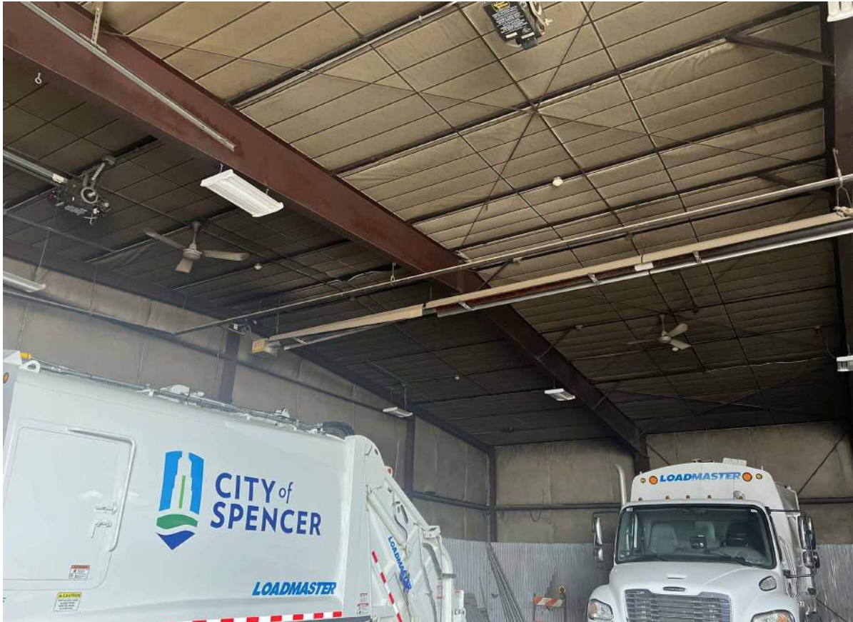
Gas Fired Radiant Tube Heaters
