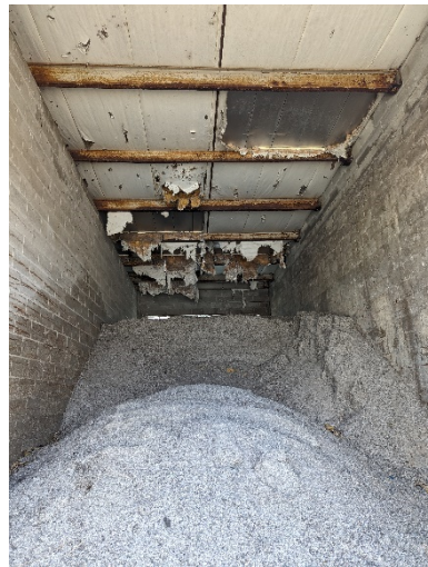
Fig 14. Failed insulation and corroding steel members
