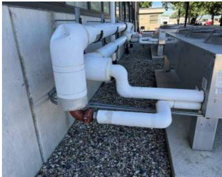
Exterior Condenser for Chiller 1
