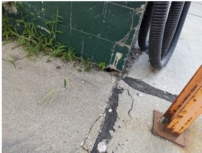
Fig 1. Void in CMU at building corner
