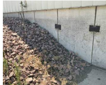
Rock Piles and Corroded Connections 1
