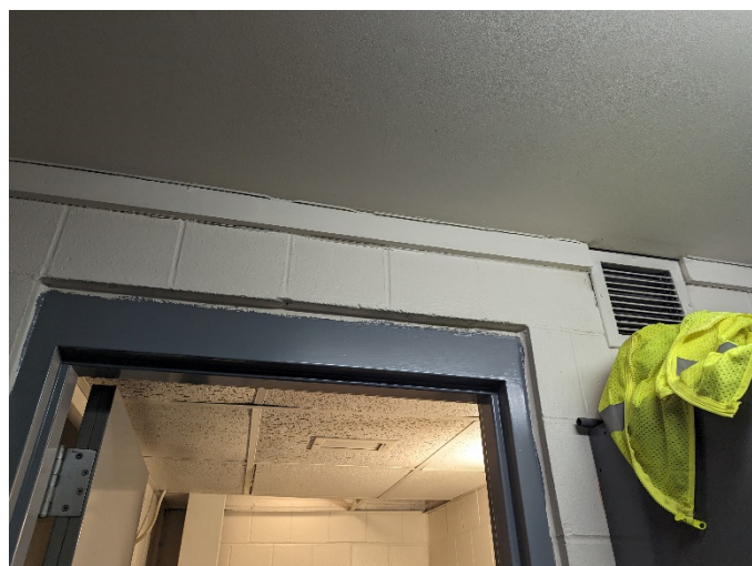
Fig 4. Crack in caulk joint at ceiling
