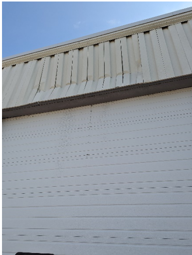
Fig 9. Damage to metal panel above overhead door
