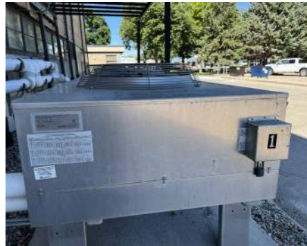
Exterior Condenser for Chiller 1
