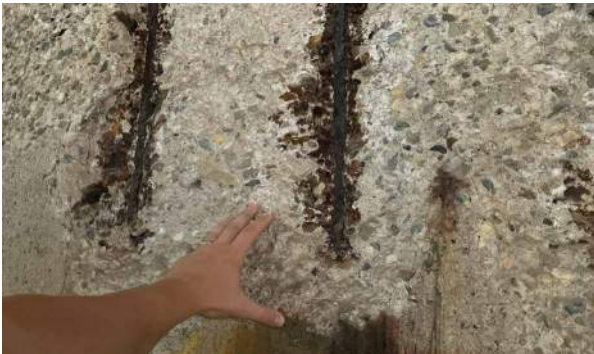
Exposed Rebar and Deterioration
