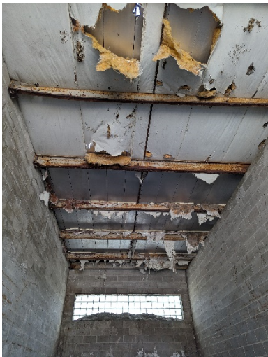
Fig 13. Failed insulation, openings in roof, and corroding steel members
