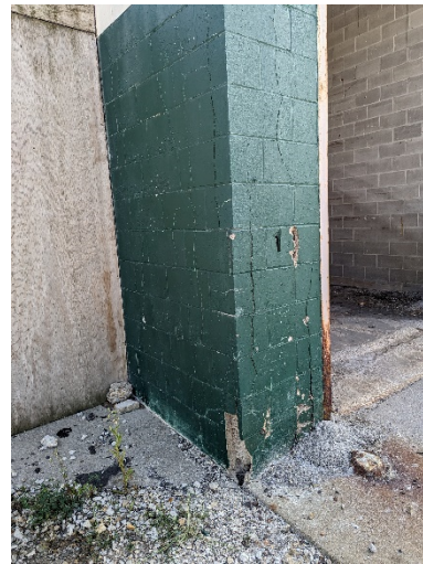
Fig 12. Cracks in CMU at salt storage building
