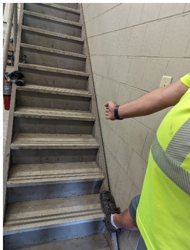
Fig 3. Separation of stair from CMU wall
