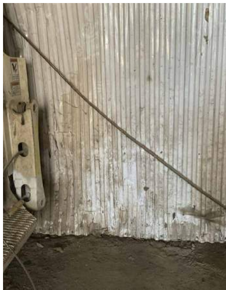
Damaged X-Bracing
