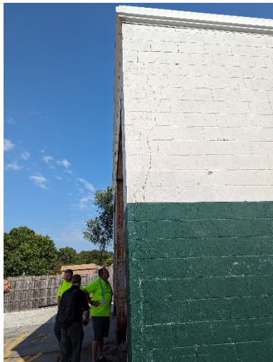
Fig 11. Cracks in CMU at salt storage building
