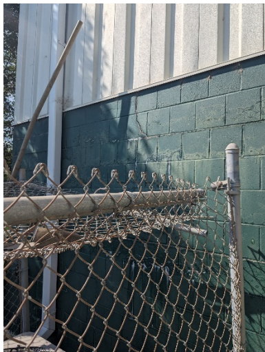
Fig 5. Efflorescence and water infiltration at CMU wall
