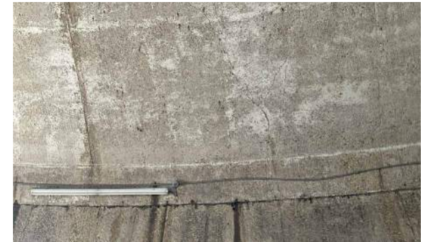
Cracks in Concrete Roof
