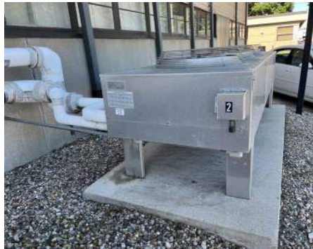
Exterior Condenser for Chiller 2
