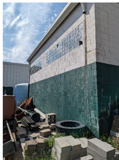
Fig 16. Damage at glass block windows and missing downspouts
