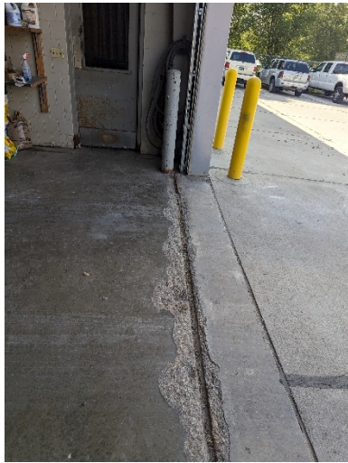
Fig 7. Spalled concrete at base of overhead door
