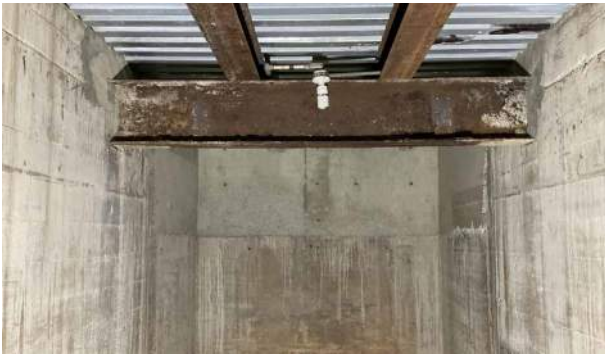
Rusted Floor Beam and Deck
