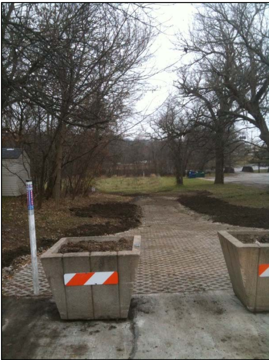
75 th and Wilshire Erosion Control Project
