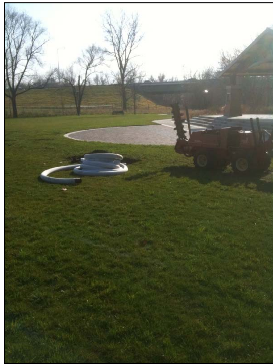
Colby Park Drainage Repair
