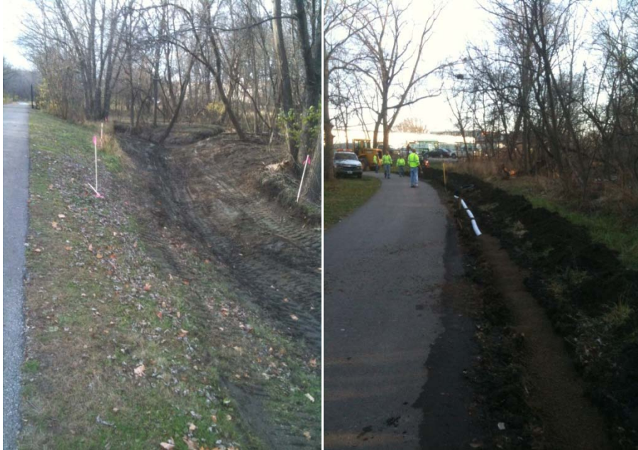
Trail Drainage – before and after
